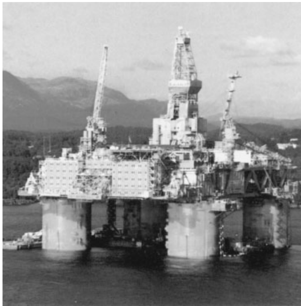
Figure 12 Demands of the superstructures of offshore oil rigs in high humidity and water exposure are met with 5454, 5086, and 5083 Al–Mg alloy welded construction.
